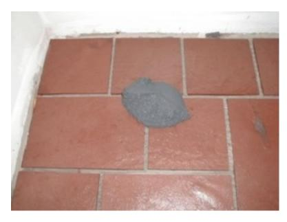
In this photo, you can see I scooped out a glob of grout from the bucket. A 4-inch drywall taping knife is a great tool to use for this purpose. The grout you see in this photo is just about enough to fill the grout lines that are visible in the photo. You only want to apply as much grout as you can spread in an area about 2 feet by 2 feet square. You can always scoop more grout from the bucket, so there's no need to make a huge pile in one spot and move it around.
