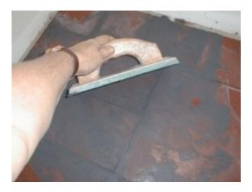
You want the top of the grout at each joint to be flush with the top of the slate or tile on either side of the joint. This will not always be easy as some slate can be thicker than others. You'll see how the rubber float controls this fairly well as you glide it across the slate. Note in the photo, how almost all of the excess grout has been removed from the slate.
