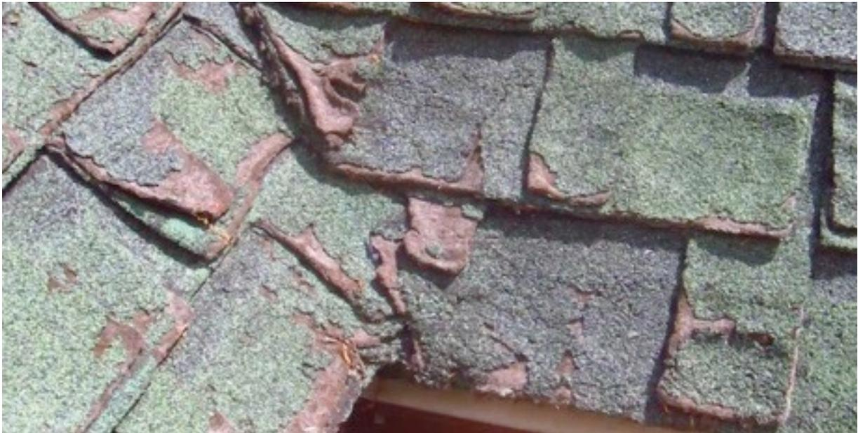
My house roof has a steep 12 / 12-pitch roof and gravity finally won the battle as the asphalt cement used to bond the lower layer to the upper layer of some of the shingles lost its adhesive power.
